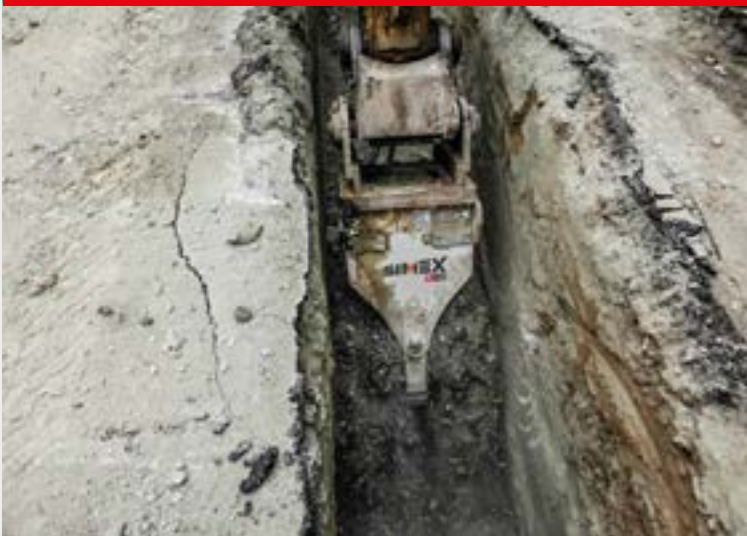
NARROW-SECTION TRENCHING
