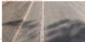
RESURFACING AFTER LAYING FIBRE OPTIC CABLES
